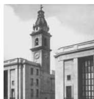
2. Torino Steeple, San Carlo Church
