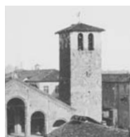
1. Milano Steeple, Basilica of Sant' Ambrogio
