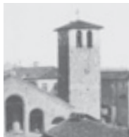
1. Milano Steeple, Basilica of Sant' Ambrogio
