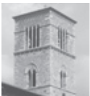
16. Terni Steeple, San Francesco Church
