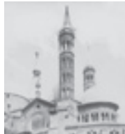
8. Padova Steeple, Basilica of Sant' Antonio
